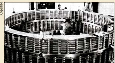
A coil of the huge superconducting magnet built at Argonne for the 12 ft bubble chamber, a pioneering application of superconductivity.
